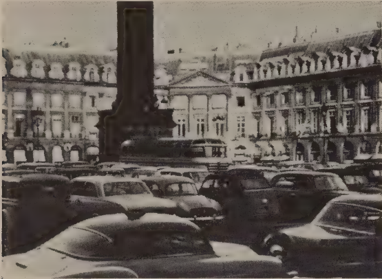
25 '... buildings seem to rise from a plinth of cars' (Place Vendôme, Paris).
